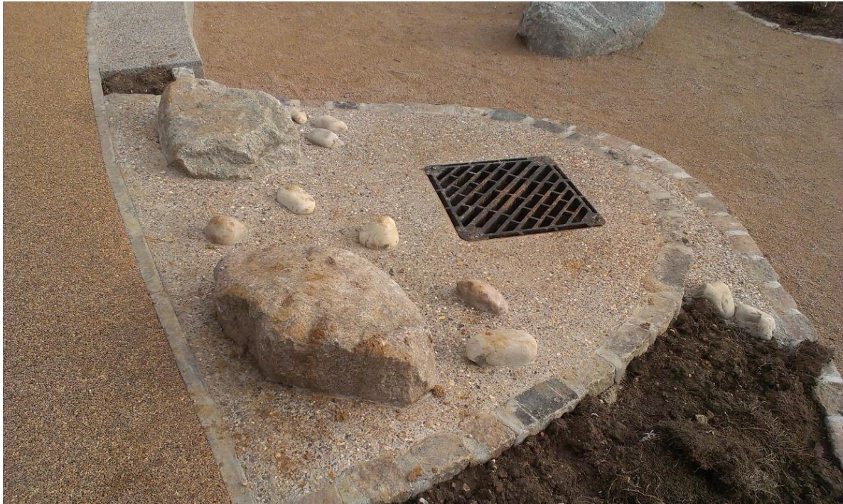
Fig. 23 Photo showing drain cover close to main inflow
